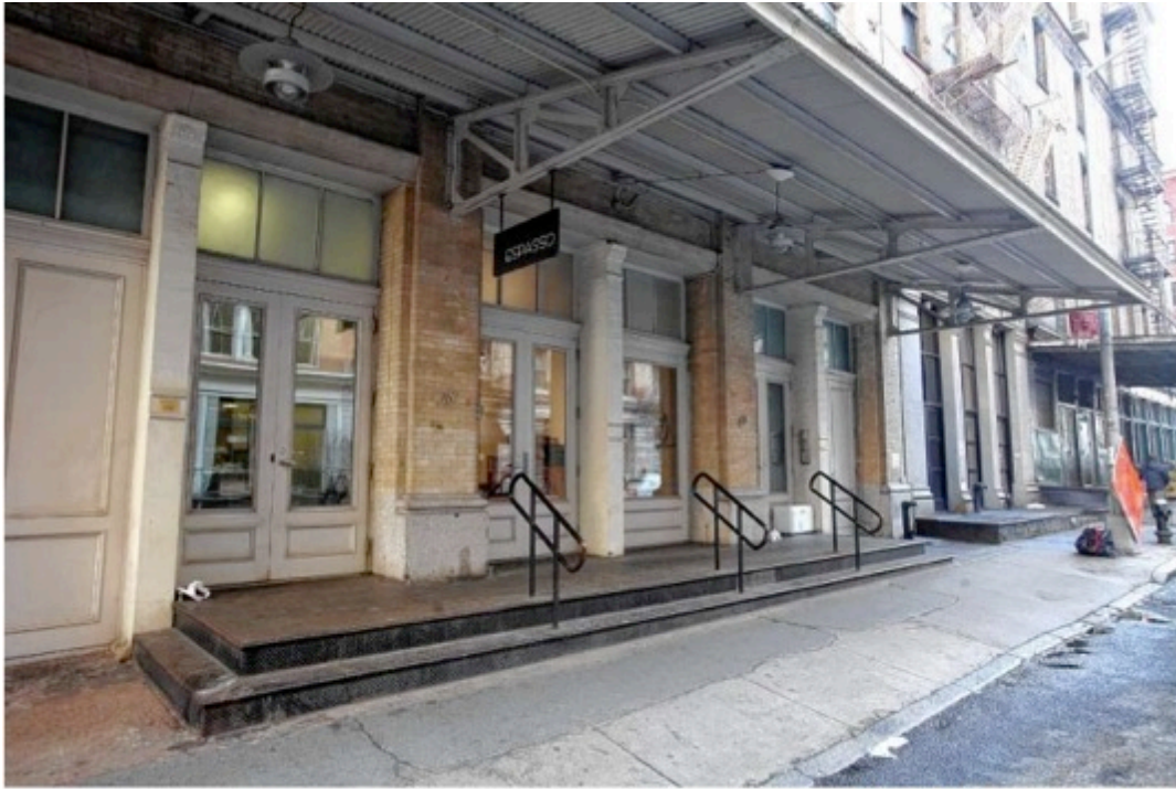
Exterior of Espasso at 38 North Moore St.
